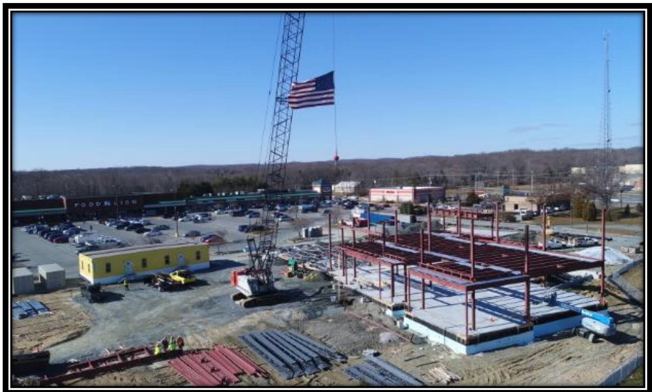
New North East Library construction site in February 2020.
