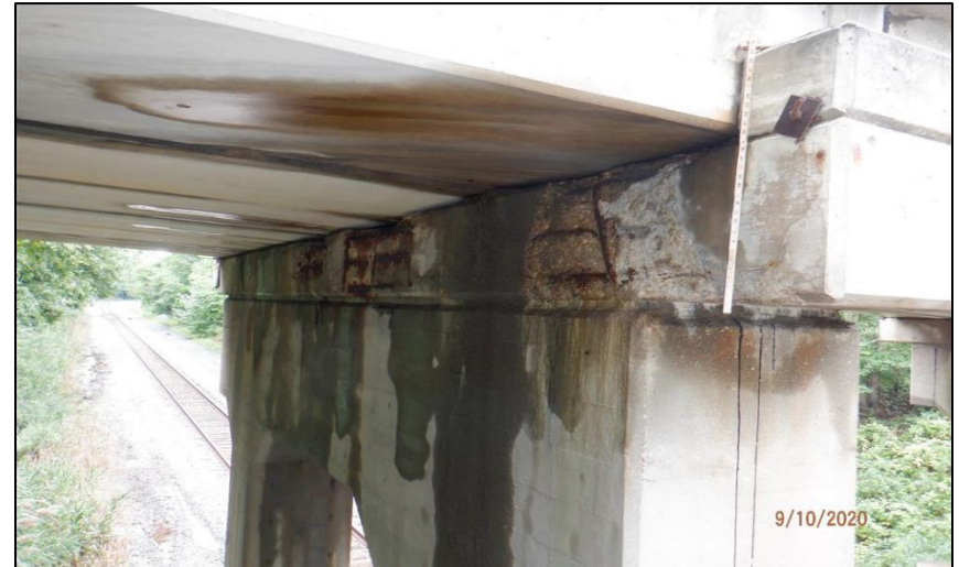
CE0055 Existing Conditions
