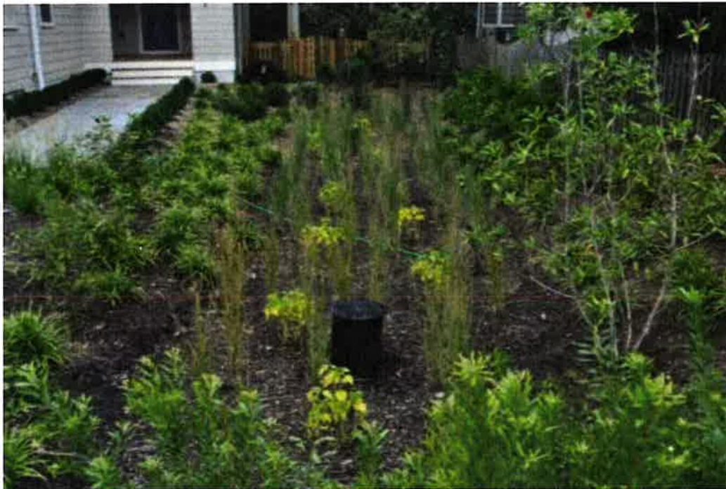
Figure 5. Rain garden to hold and treat stormwater.
