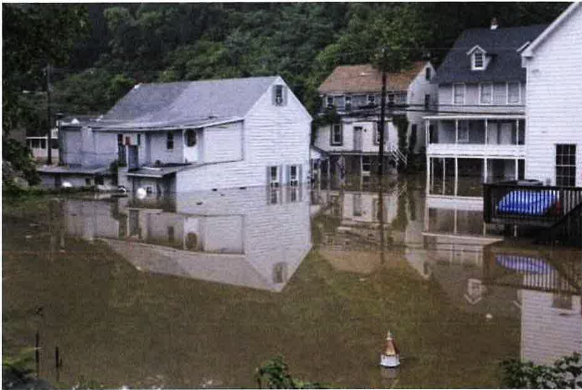
Figure 2. Flooding in Port Deposit from Tropical Storm Lee. (Photo: Cecil County Department of Emergency Services)
